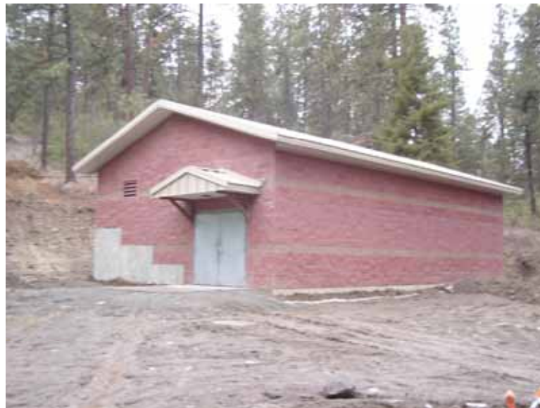
West Drive Booster Station
