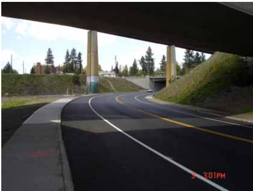
Westside Water Main Project – Inland Empire Way
