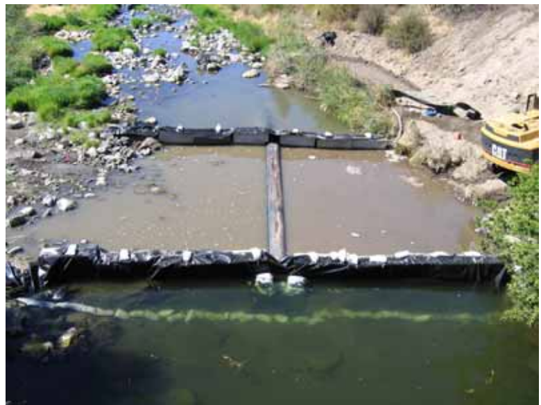
Marne Bridge Siphon Replacement During Construction
