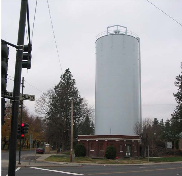
14th Avenue and Grand Boulevard - Elevate Standpipe
